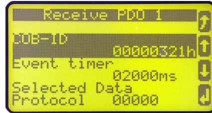
Figure 2-24: Display screen - Receive PDO 1 for changing the set point
